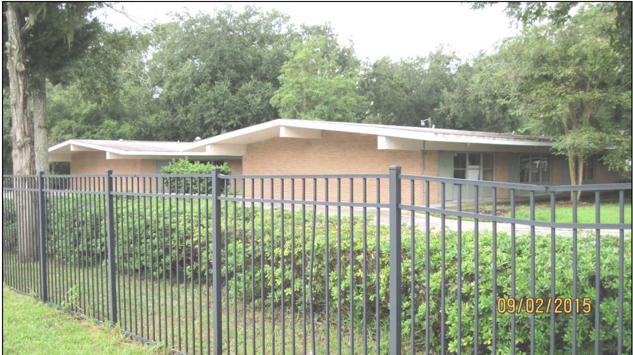
Daycare and classroom space existing on site, along Spring Park Road.
